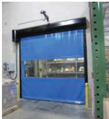
FIGURE 3. LiteSpeed HZ high-speed door is UL listed for hazardous-rated environments. The door has a Class II, Division 2 listing from UL, carrying a Group Code G and Temperature Code 6, which means it can safely operate in facilities where combustible dusts such as flour, grain, wood, plastic or chemicals are not normally in the air but can be present
