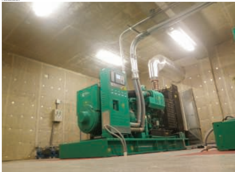
FIGURE 6. Acoustiblok soundproofing material is a thick, advanced sound barrier material that is placed between a noise source and the noise receiver. The viscoelastic, flexible, dense polymer material with a high-density mineral content contains no barium, lead or asbestos
