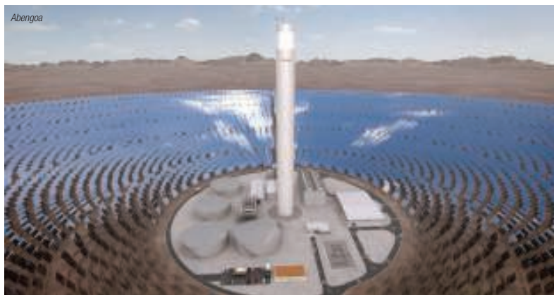
FIGURE 3. Abengoa is developing South America’s first CSP plant in Chile. The plant will use an advanced storage system enabling it to generate electricity for up to 17.5 h without direct solar radiation
